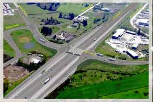
New LaBree Interchange Est. Completion 2009
